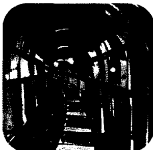
TUNNEL ENGINEERING Tunnelling Operations.
