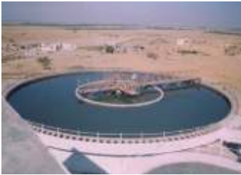
Water Treatment Works at Shirbhavi
