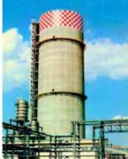
Jagdishpur Filling Tower
