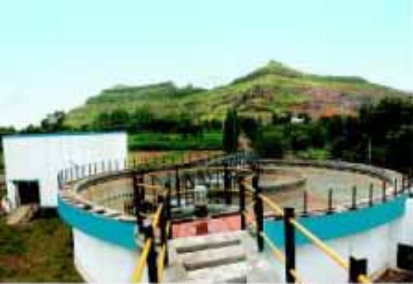
Undale Water Treatment Plant
