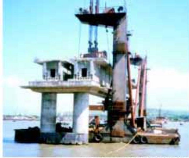
Floating Gantry for Erection of Box Girder
