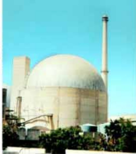
Rajasthan Atomic Power Project, Kota
