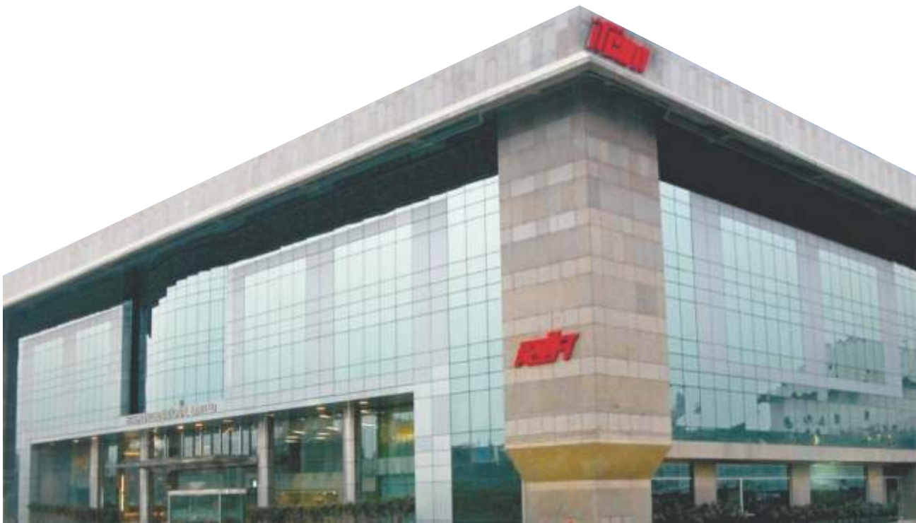
Corporate Office Building of Irrcon at Saket, New Delhi
