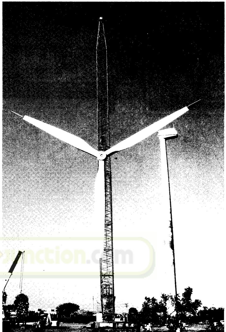
Erection of wind turbines with self assembly state of the art cranes
