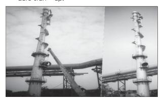
b) The following flare system has Derrick support, 45mtr height, 80" and 48"stainless steel Tip and FFG panel for auto start - up and PLC Based Controller.
