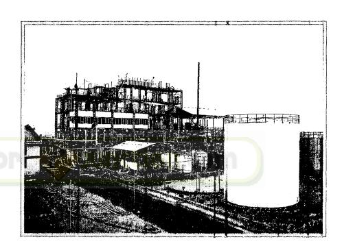
A 13,500 TPA Acetic Acid and 3,000 TPA Ethyl Acetate manufacturing unit, the Company has now commissioned new projects for the manufacture of 4,500 TPA of Acetic Anhydride, 2,100 TPA of Para-amino Phenol and 5,100 TPA of Sodium Sulphate.
