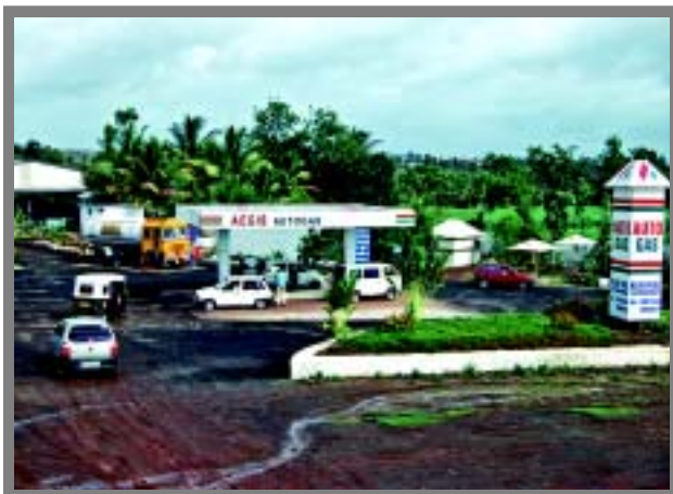
Aegis Autogas Station at Kolhapur
