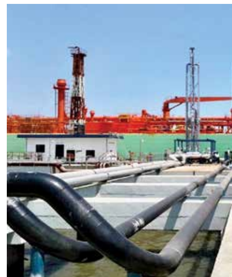
Newly installed LPG unloading arms at MbPT
