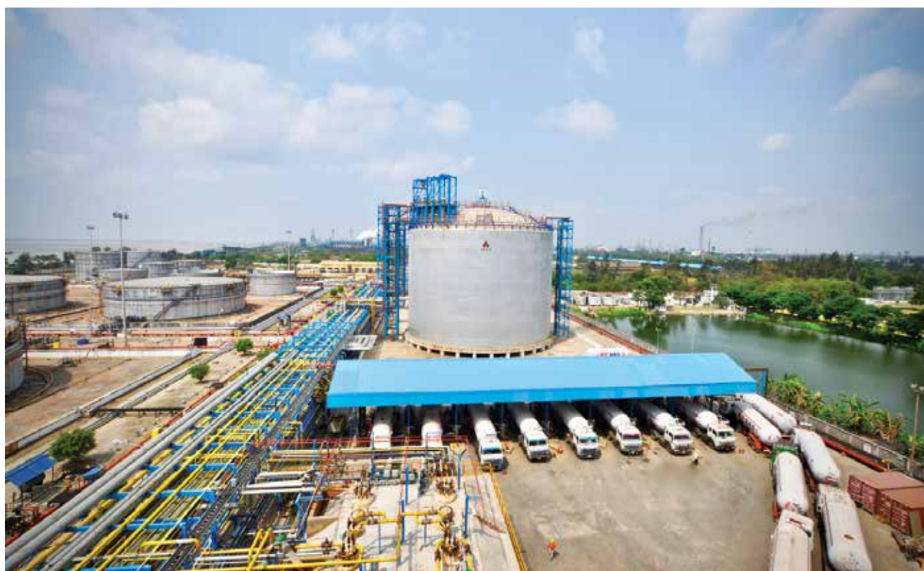
Newly commissioned Haldia LPG Terminal
