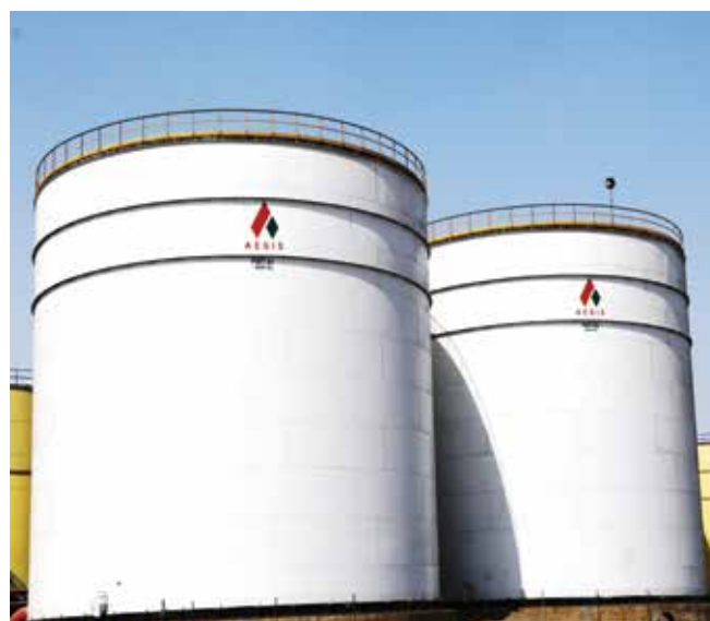
Newly commissioned tanks at Kandla Liquids Terminal
