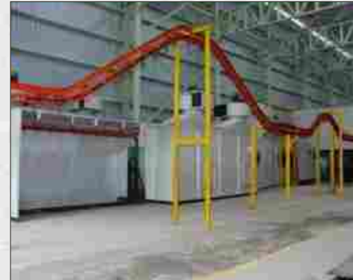
Pre-treatment Plant at Jejuri
