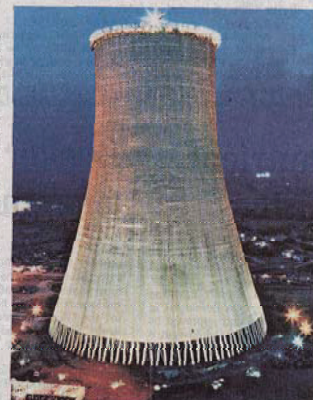
Natural draft cooling tower at the Kalsindh power plant of Rajasthan Rashtriya Utpadan Nigam Ltd., in Rajasthan, claimed to be the world's tallest (202 metres).
