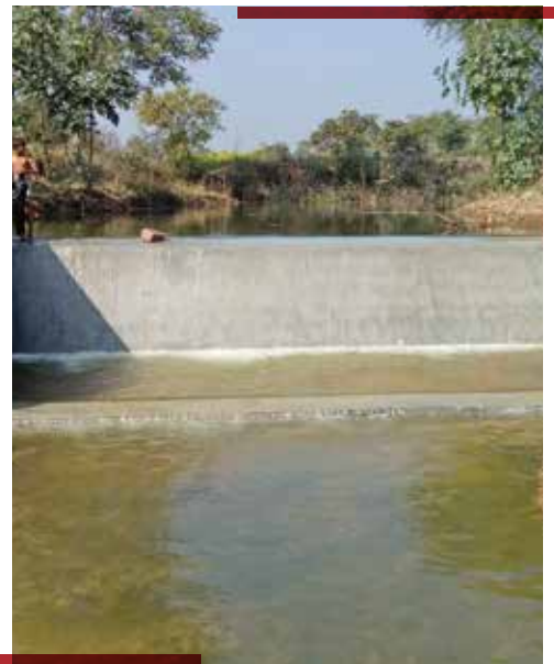
Construction of check dam with 1.5 lakh CUM storage capacity, benefiting 75 farmers and 570 acres of farming land
