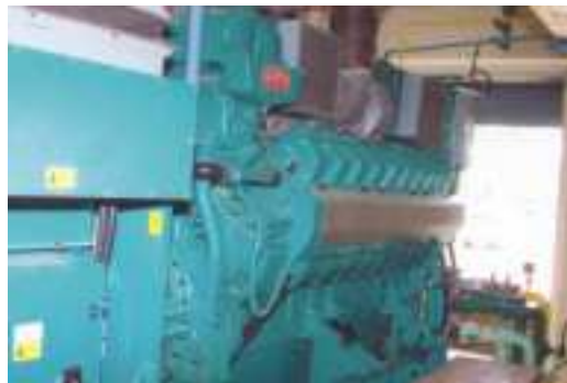
1750 kW QSV 91-G lean-burn natural gas based generator set at Raghav Industries Limited, Ankleshwar
