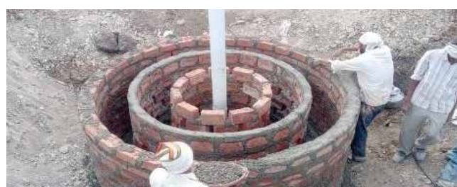
Jal Sanrakshan, recharge shaft for groundwater development for sustainable farming at Nidhona village, Aurangabad, Maharashtra
