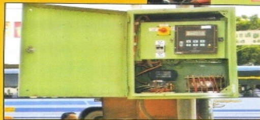
Installation of EPIC's Power Savers with REMS (Remote Energy Management System) in Madurai, Karnataka
