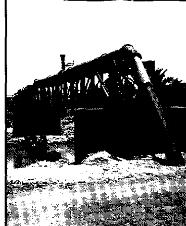
Pipe Structural Cross-Over for HPL (Haldia) Raw Water Pipeline (DN600 pipeline)
