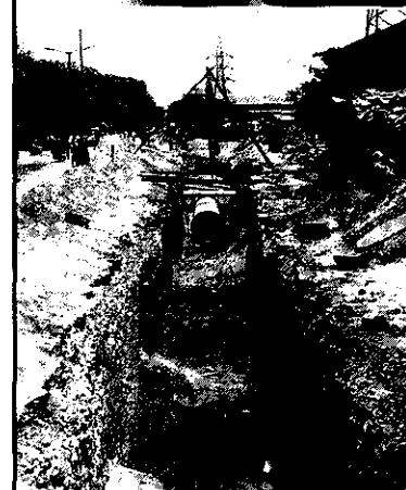
Sewage Pumping Main for Ahmedabad Municipal Corporation (DN 1000 pipeline)
