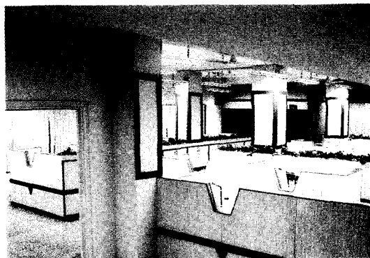
Partitioning using E-Board
