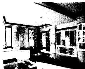
False Ceiling using E-Board
