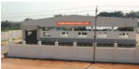
Unit 4 Location: Mysore, Karnatka Establishment: 2005 Products: Rear Fender Assembly Land Area (Sq. Mtrs): 4,014
