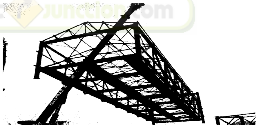
Design, fabrication, supply & erection of pre-fabricated steel roof structure including roof portals, purlins, sheeting etc. for stations at Noida, Anand Vihar & Akshardham Station for Delhi Metro Rail Corporation Ltd.
