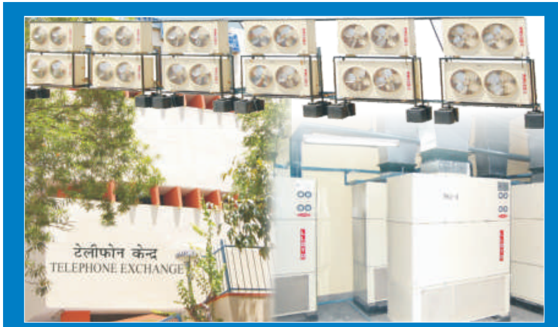
High Sensible Packaged Airconditioning Unit for Telecom Sector
