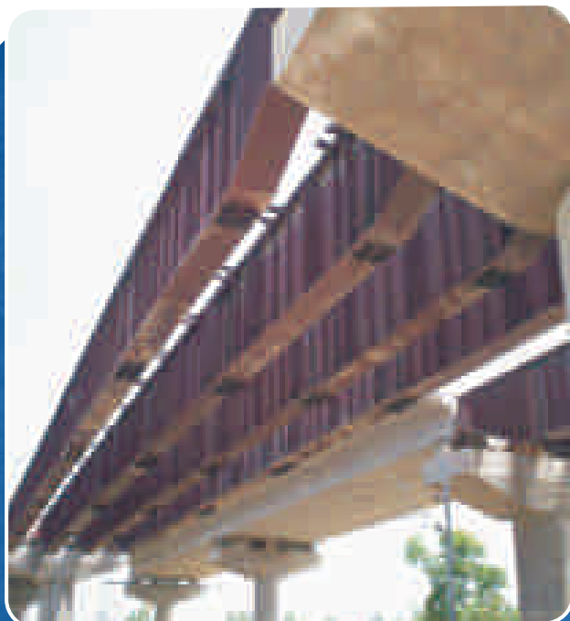
Complete fabrication and installation of 55m clear span Railway Over Bridge at Moradabad-Bareilly highway
