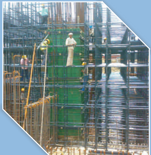
Column erection at Koradi, Nagpur
