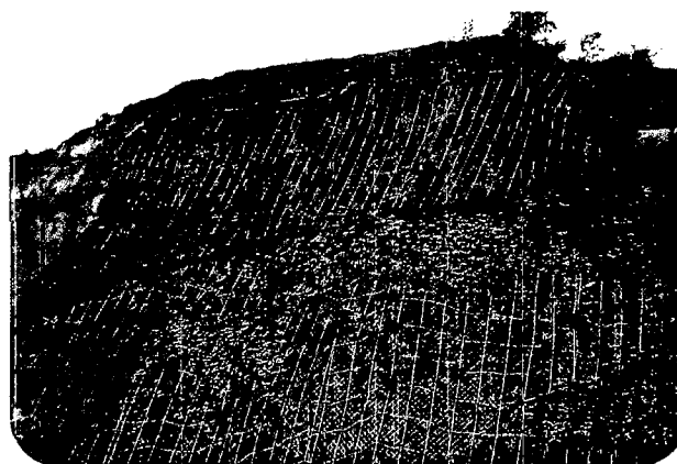
Roads : Rock fall protection net prevents loose rocks from falling on rail tracks and roads
