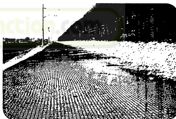
Railways : Railway track-bed stabilisation
