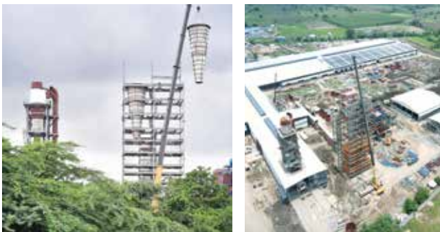
Cyclone installation at Greenfield MDF board manufacturing unit, Vadodara, Gujarat
