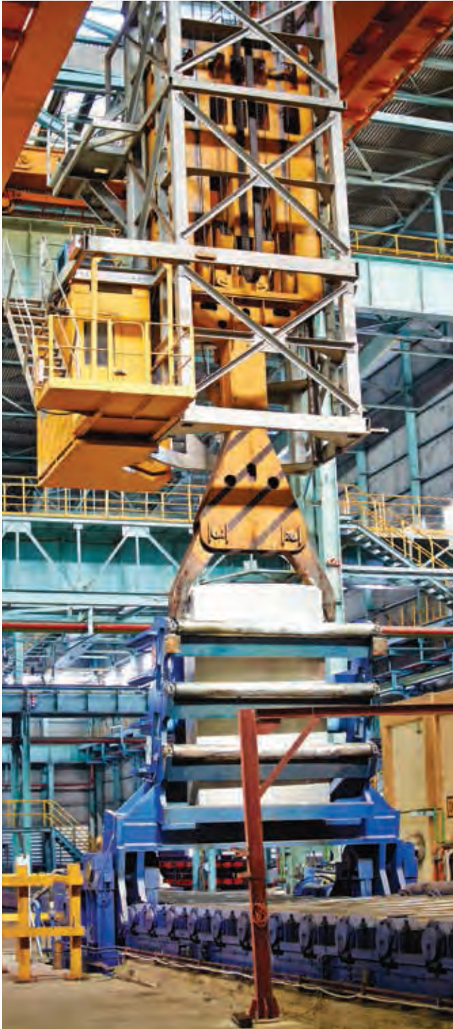
Aluminium FRP plant in Hirakud, Odisha
