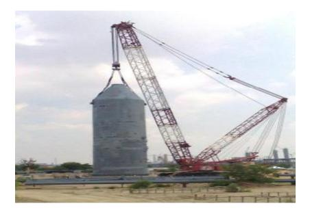
Water seal drum equipment supplied to HMEL Bhatinda having Design Pressure 3.5Kg/cm2; Design Temp: 220°C, MOC SA516GR70, Shell Dia is 7700mm, Length is 12500mm, Shell Thickness is 20mm, and Weight is 229MT.
