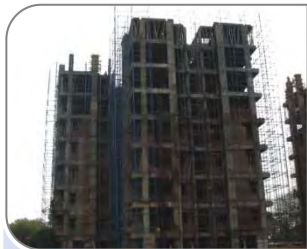
Maytas executing housing project in Kanpur
