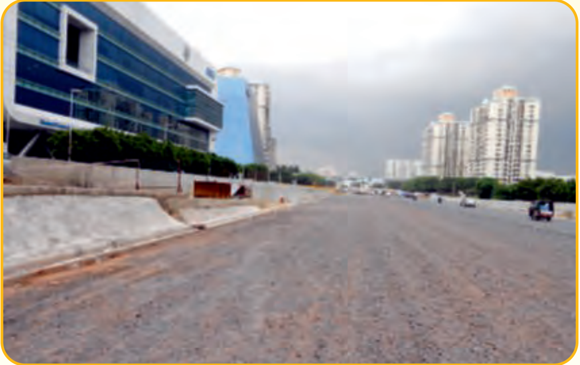
Dense Bituminous Macadam (DBM) layer completed at Cyber City area at DLF Road Project, Gurgaon
