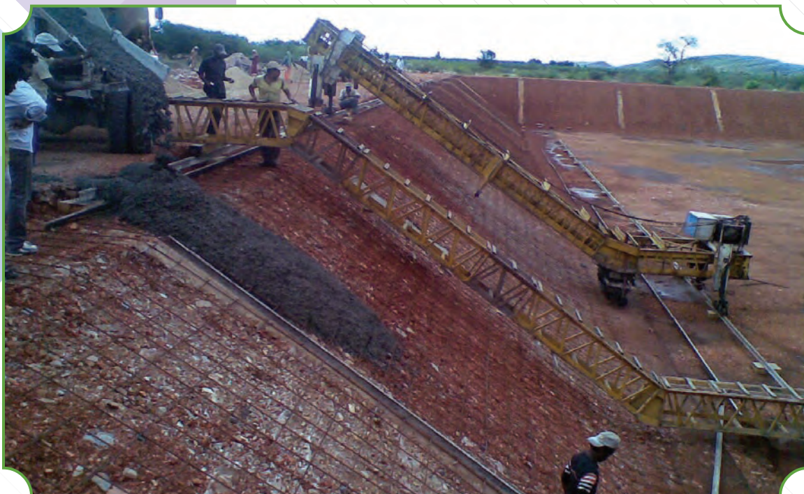
CC lining work in progress at main canal as part of Lingala irrigation project in Kadapa District of Andhra Pradesh
