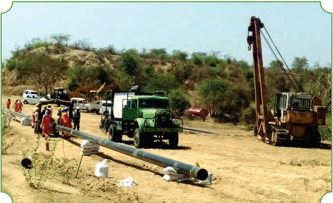
Mainline welding works for 12 inch pipeline in progress for natural gas pipeline project of Gas Authority of India Limited (GAIL) in Gujarat
