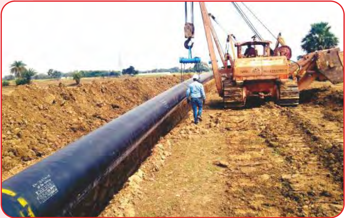
Phulpur-Haldia Pipeline Project Lowering at Chainage 313, Bihar
