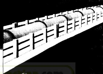
A World Bank funded Project for drainage of Hyderabad Municipal Water Supply and Sewerage Board, using 1,800mm dia NP4 class R.C.C. Pipes, lined with high Aluminia Cement. Lenght - 5 Kms Project cost Rs. 13 crores. Thousands of Kilometers of R.C.C. Pipeline have been laid by IHP across India, Pakistan, Burma & Sri Lanka.
