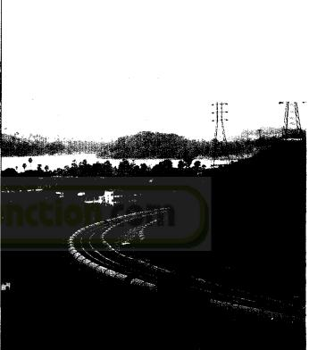
IHP's steel pipes widely used by B.M.C. for augmenting water supply to Mumbai city. About 129 Kms. of Pipelines in various diameters of 450mm to 3658mm. and weighing nearly 79,000 M.T. are supplied by the Company.
