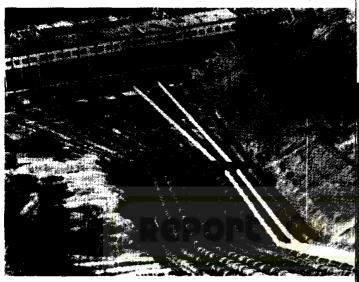
Penstocks of 2438mm dia. ranging in thickness from 16mm. to 30mm. weighing 21194 M.T. are installed at Sharavati Hydro-Electric Project.
