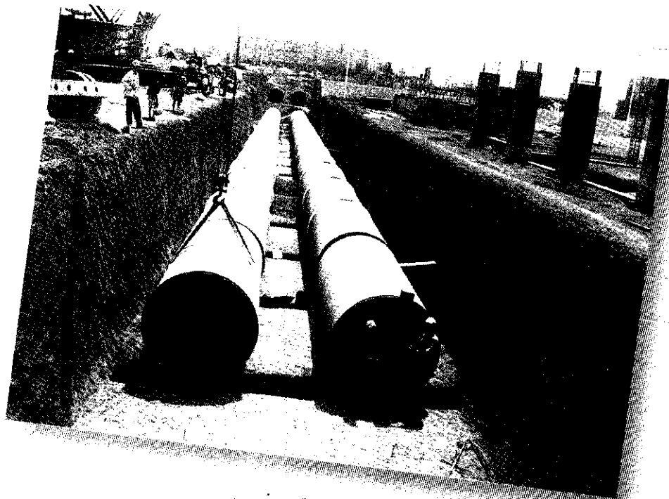
1800 mm dia BWSC co circulation pipeline at combined cycle power M/s BSES Ltd. near K Andhra Pradesh.
