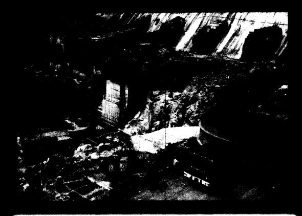
4480mm & 7800mm dia Penstock pipes erection work is in progress for Almatti Dam Power Project in Karnataka State. The total tonnage involved is 1230 M.T., valued at Rs. 486 Lacs.
