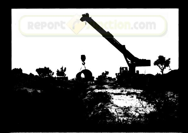
900mm dia. 24 kg/cm2 pressure PSC pipe laying in progress for the 42 kms. long water supply pipeline under Churu-Bissau Project in Rajasthan valued at Rs. 2613 Lacs.
