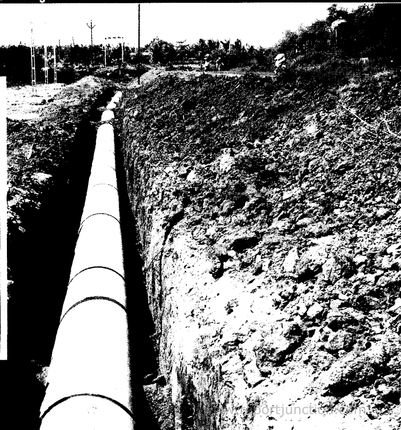
700 mm dia Bar Wrapped Steel Cylinder pipeline for Gujarat Water Supply & Sewerage Board
