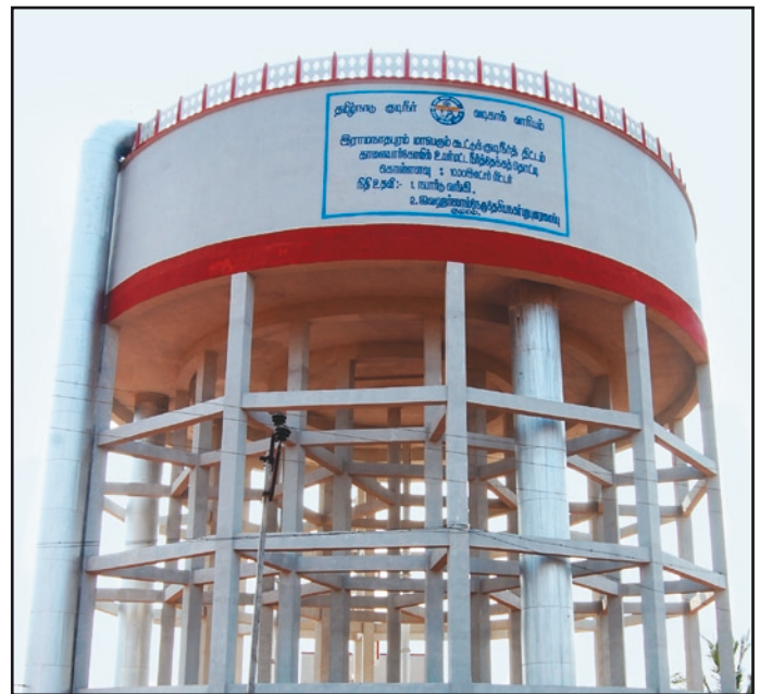
10 Lacs litre capacity overhead tank for Water supply scheme for Ramanathapuram, Sivagangai and Pudukkottai Districts
