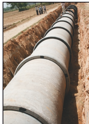
2000 mm dia PSC pipe line for U.P. Jal Nigam Ghaziabad
