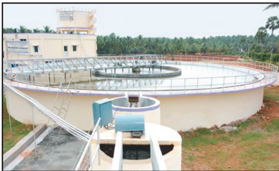
Clarifloculator at Combine Water Supply Scheme to kurichi, kuniamuthur and kinathukaavu in Coimbatore District
