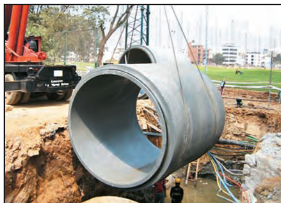
2400 mm dia R.C.C. NP-3 class pipe with polyurea lining for the sewerage work contract S2B for BWSSB, Bangalore
