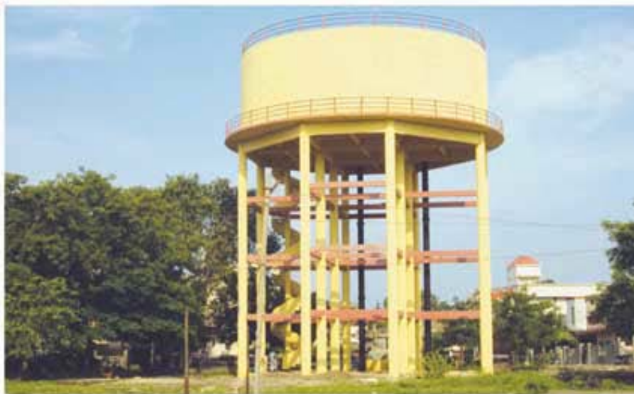
Elevated Storage Reservoir of 9.15 Lakh Liter Capacity
