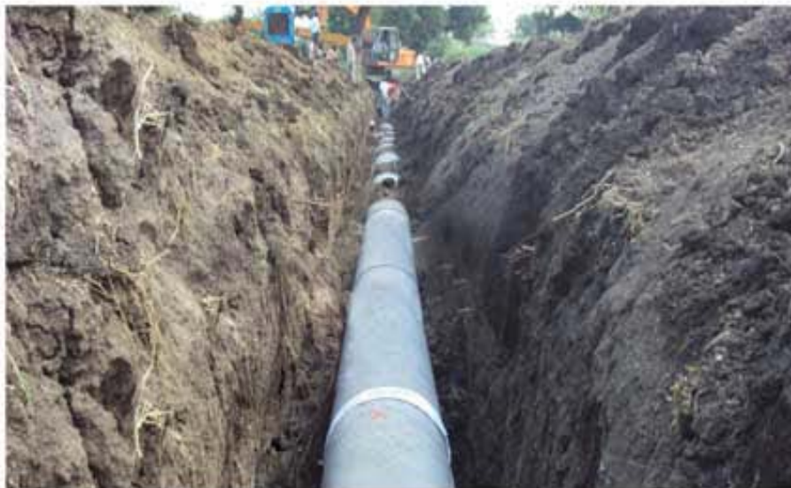
600 mm Dia Prestressed Concrete Cylinder Pipe Line (49 KM)
