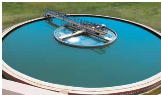
Clariflocculator at Dharmavaram Water Supply Scheme
