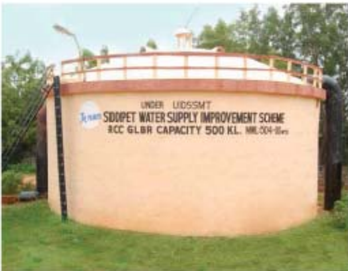
Ground Level Balancing Reservoir of 5 Lakh Liter Capacity.
