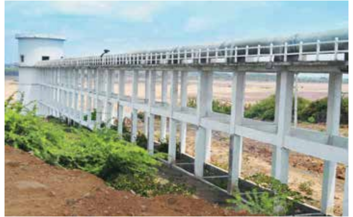
Intake Well Cum-Pump House in River Godavari for Bhadrachalam Water Supply Scheme
