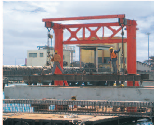
Beam erection by gantry at Tuticorin, Tamilnadu
