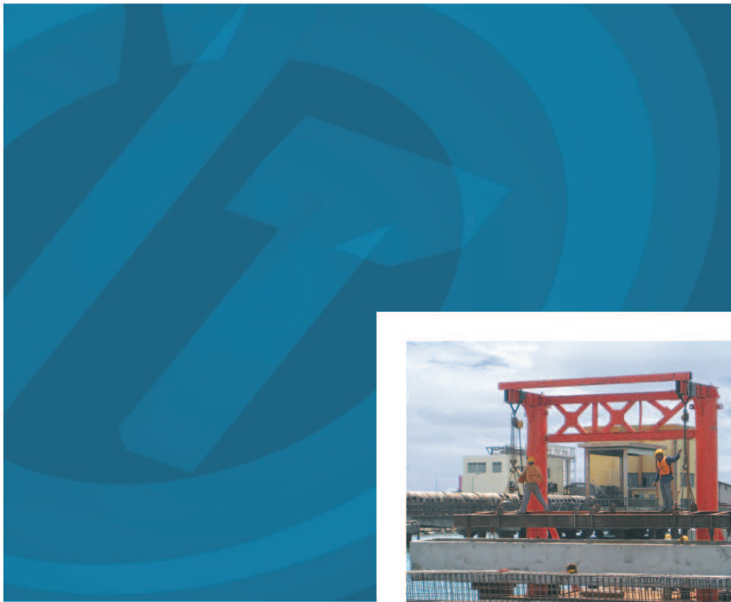
Beam erection by gantry at Tuticorin, Tamilnadu
