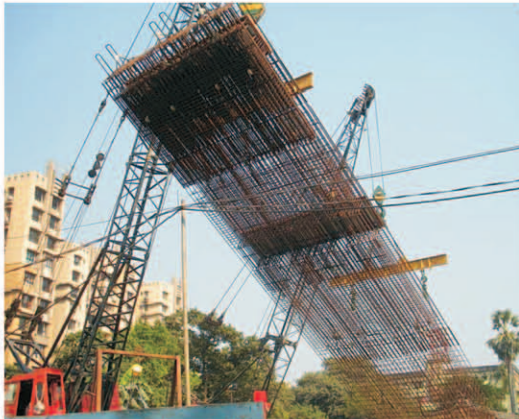
Diaphragm wall cage lifting at Subhas Sarobar at Kolkata
