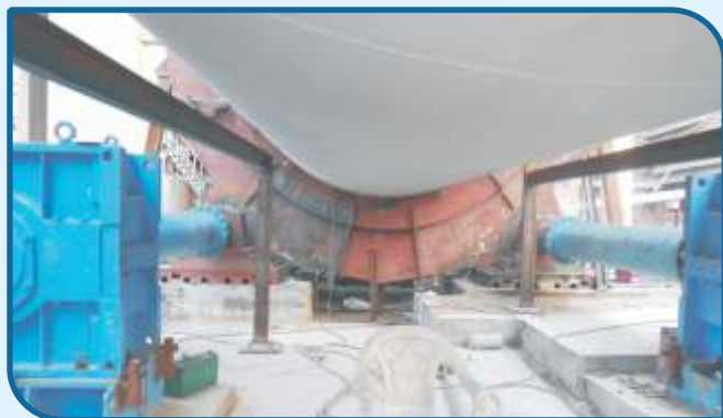
Hot Air Recirculation in line-1 IKN cooler installed as part of the Company's Power Saving Initiative
