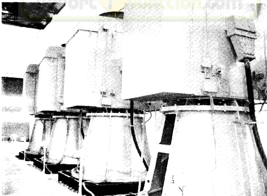
'Jyoti' make 1200 VM Battery of Pumps for Krishna Bhagya Jal Nigam Ltd. at Indi Irrigation Scheme, Bangalore : Motor Rating 2100 KW, Discharge 4.97 m 3 /sec, Head 34.18 Metres
