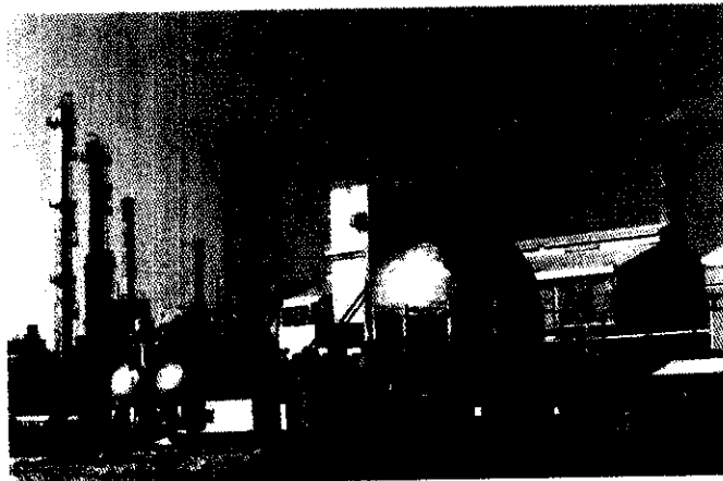
A general view of Ammonia Plant at NFL Panipat
