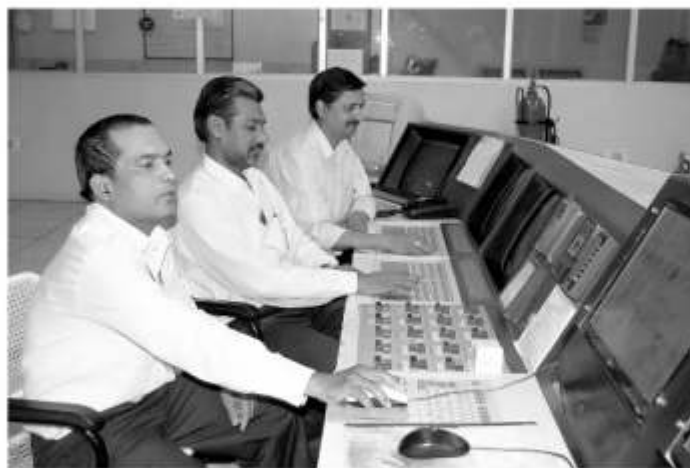
Employees working on digital control system (DCS) in Vijaipur Plant
