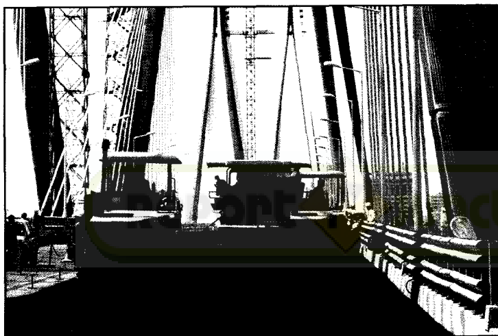
Providing asphaltic wearing coat on Bandra Worli Sea Link Project, Mumbai
