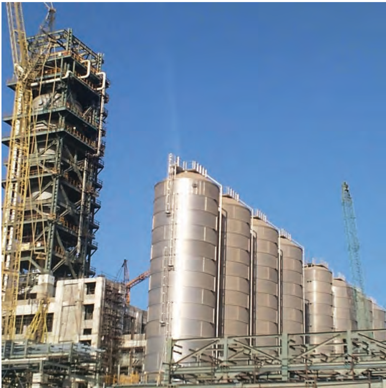
Erection of Blending Silos at Reliance Jamnagar Refinery
