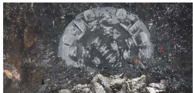
TBM breakthrough
