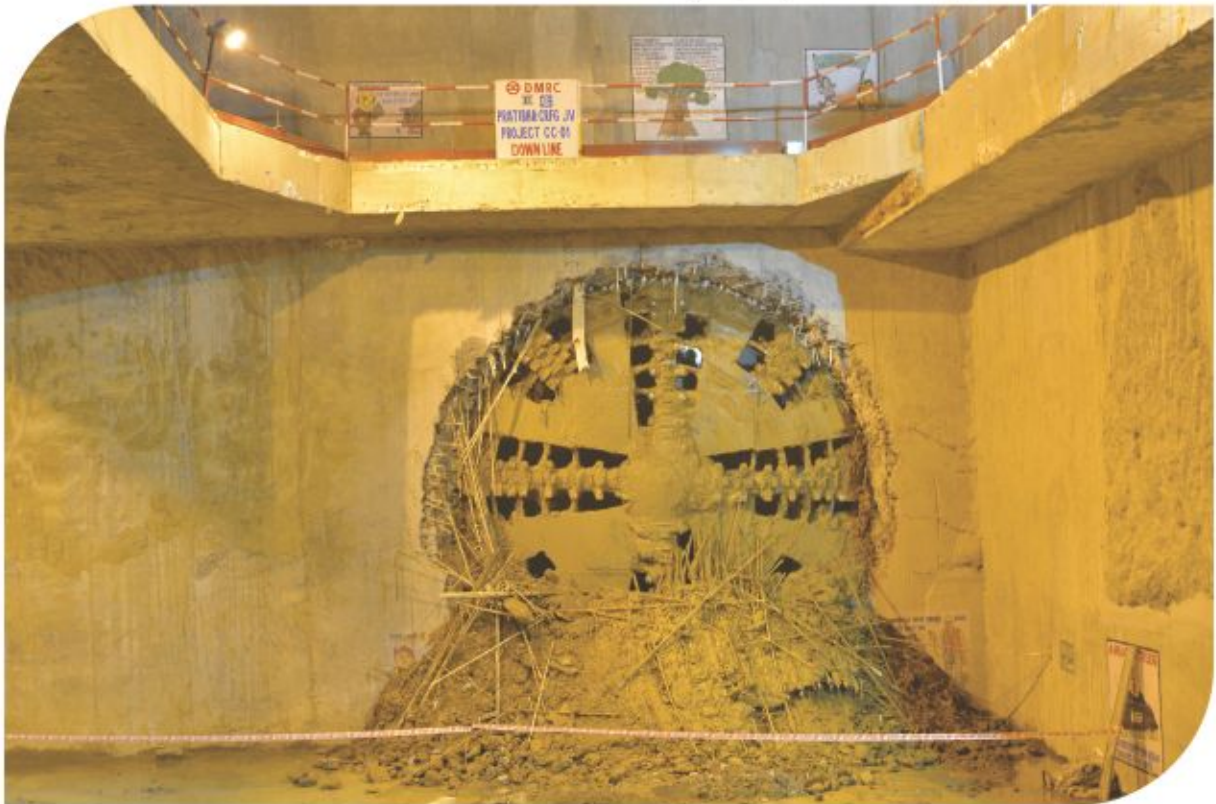
DMRC Site - New Delhi - Tunnel Day Light (Break Through)
