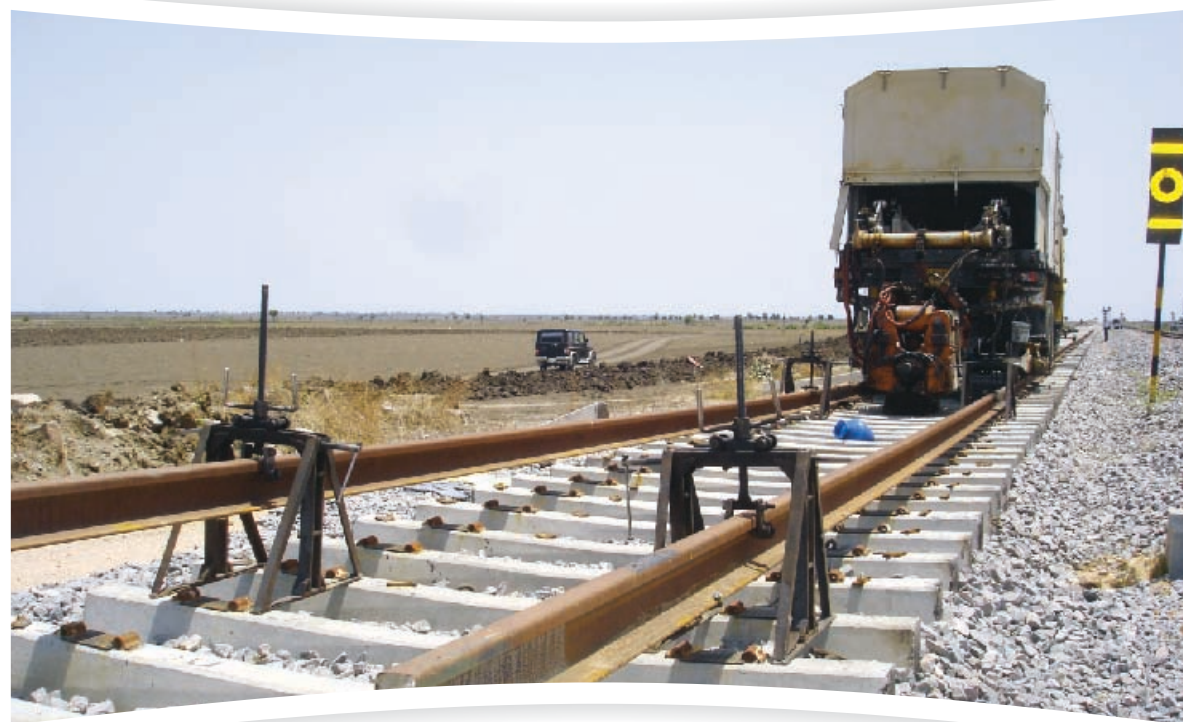
Ballast Spreading through Rail lorry in Section of Hospet - Tinaighat Doubling Project
