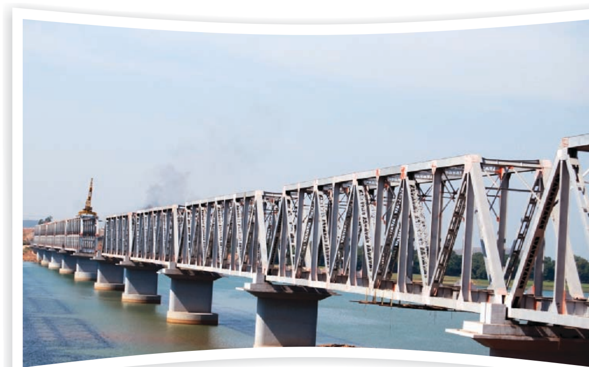
92 m steel through girder launching over river Mahanadi near Naraj in Rajatgarh-Barang doubling project.
