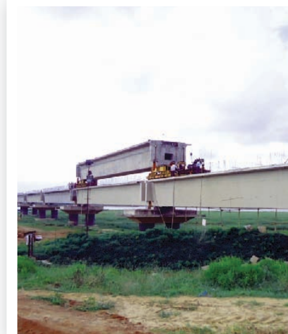
43.8 m PSC box girder weighing 650 tons launching over river Luna in Haridaspur - Paradeep NL project.
