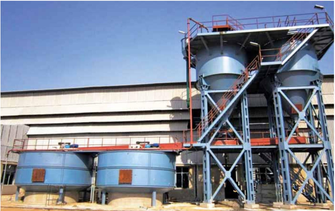
A view of Cone Tank at Kotputli Factory
